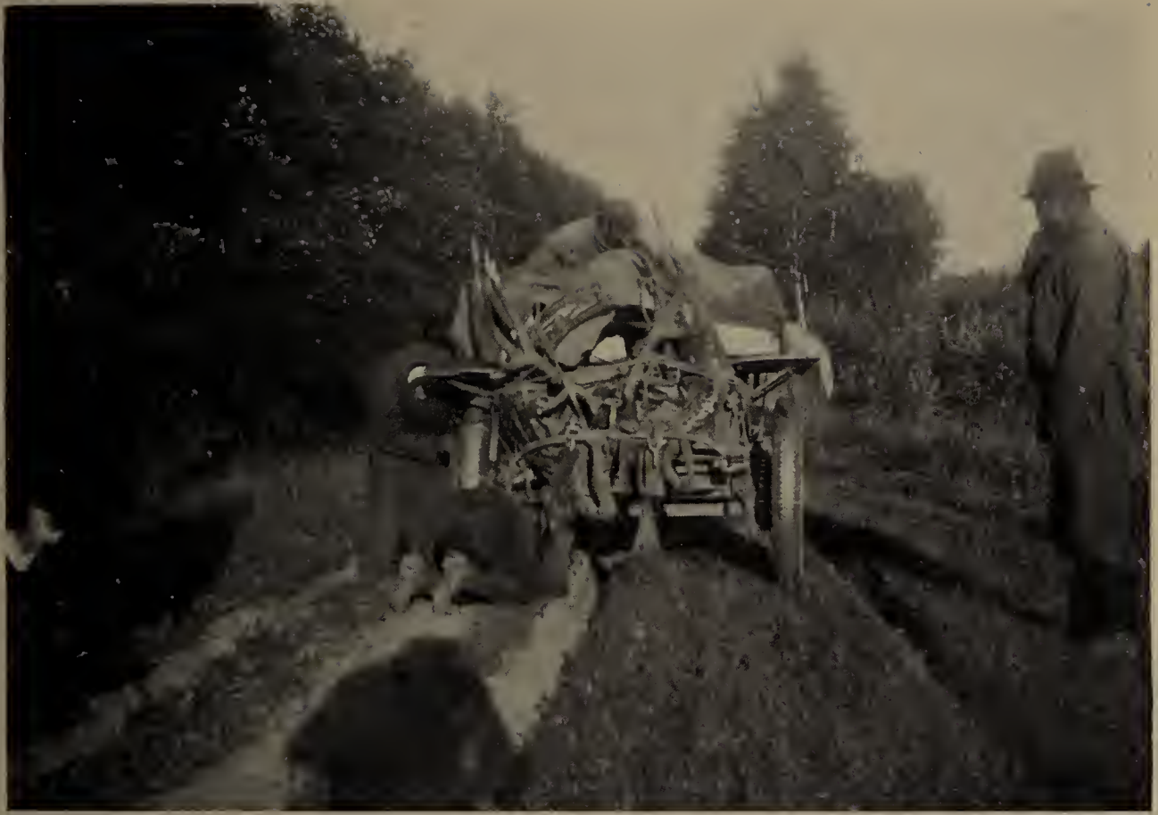
REPAIRS ON THE BAIKAL HILLS.
